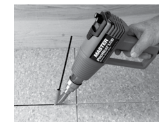
Welding Flooring Material
