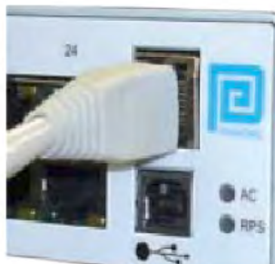
Figure 8: NIC Cable Connected*
